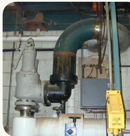
New installation of the vent pipe - proper supports are being installed
