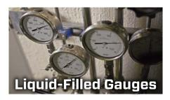
Swagelok Liquid-Filled Gauges enhance the reliability and integrity of your measuring system for long periods under extreme operating conditions by dampening vibration and lubricating the gauge movement.
