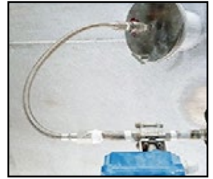
Twisting a hose or bending it on more than one plane
