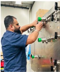
Fuel Gas Panels tap into the same available clean gas, to provide fuel to Gensets and remote power generation packages.
