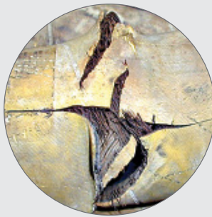
Excessive Cover Damage
