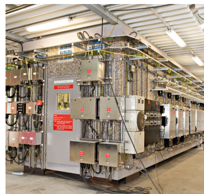
An exterior view of the analyser house.
