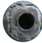
Localized Crevice Corrosion
