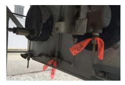
Replace leaking relief valves, valves, panels, and connections with a more leak resistant product. Consider selecting a single supplier for this application to maximize discount. A quote has been provided for Swagelok options.
