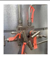
Replace all leaking connections with a more leak resistant product. Eliminate threaded connections when possible. Reduce the number of connections and leak points when possible. A quote has been provided for a Swagelok option.
