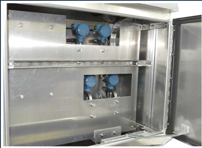
Pressure monitoring transmitters can be accessed from both front and back doors allowing for ease in calibration and equipment maintenance.
